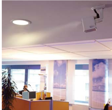
In-room spray humidification
