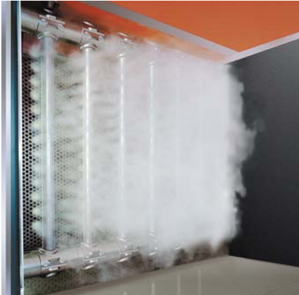
In-duct steam humidification
